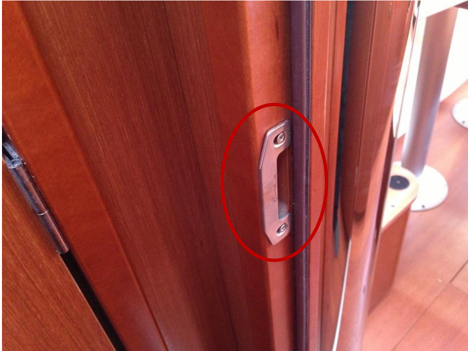
Bow cabin this door part needs to be tighten.
