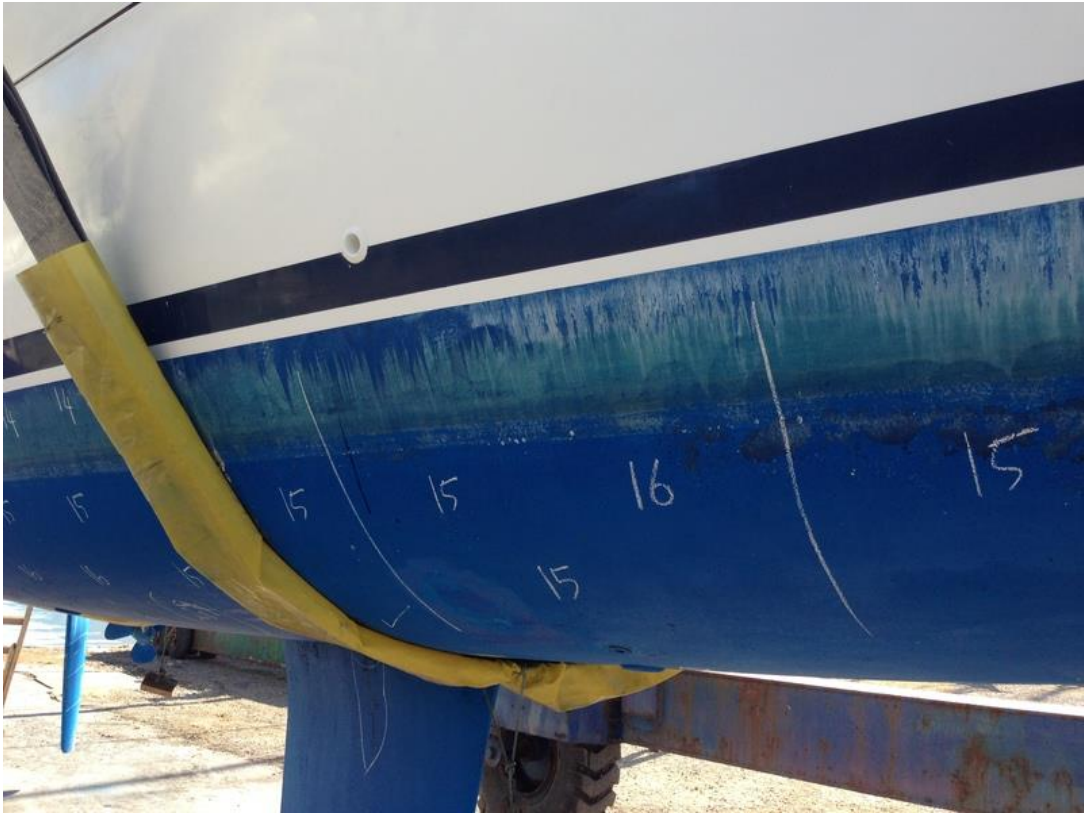
General moisture on grp was about 15%. This is acceptable level for one day standing boat on land.
