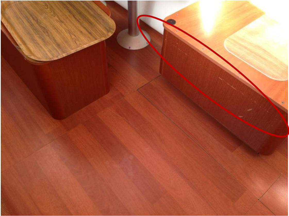
Cosmetic defects on saloon.
